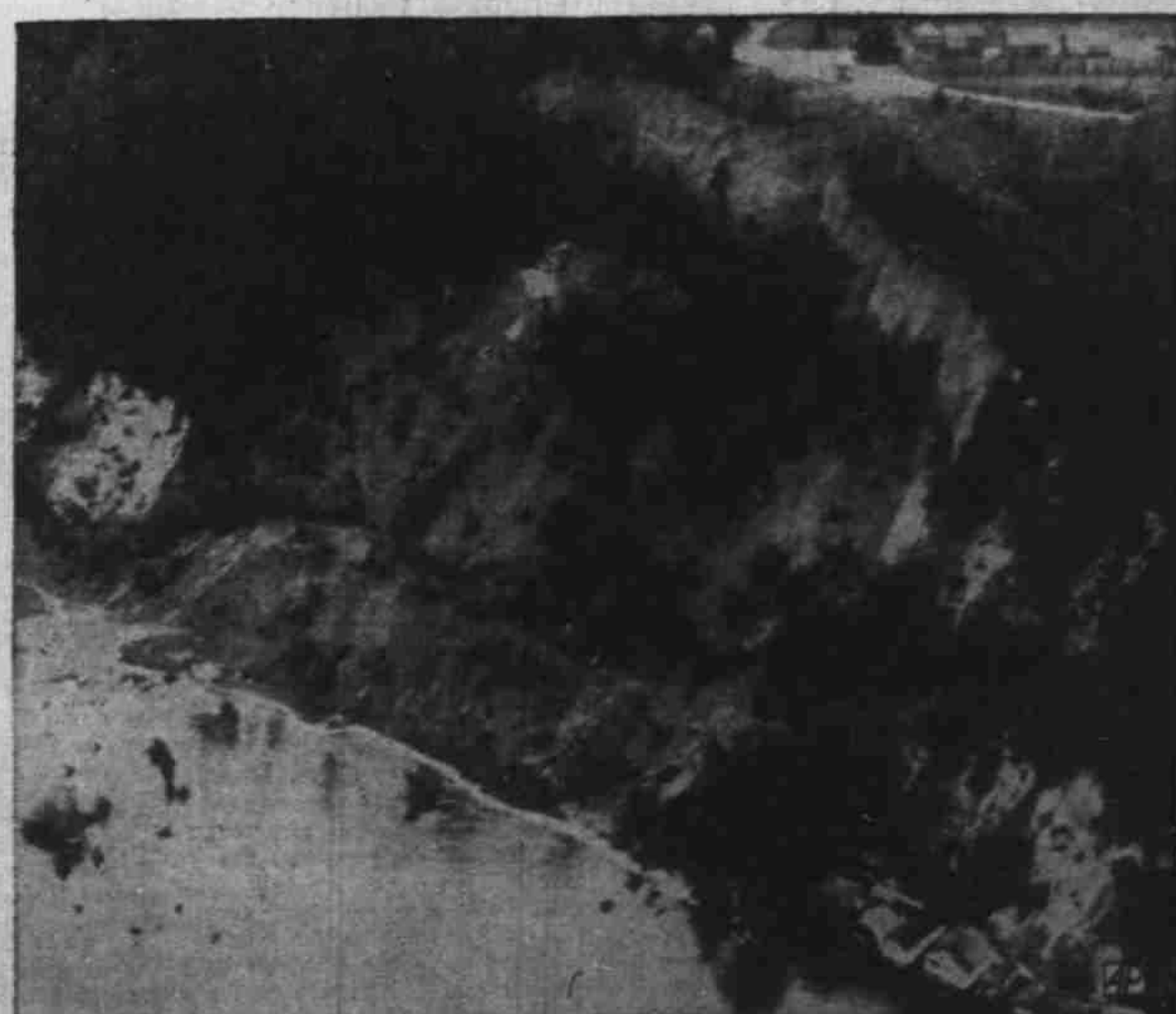
QUAKE-CAUSED SLIDE SCENE—This air photo shows where a cliff 400 feet high roared into Puget sound, barely missing the edge of Salmon Beach community (foreground) near Tacoma, Wash. Wednesday's earthquake is blamed. Old Fort Nisqually (upper right) is close to the edge of the slide. Trees protrude from what was 100-foot deep water. (AP Wirephoto).
