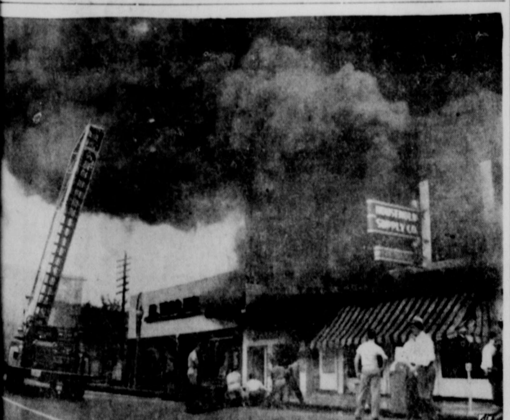
FIREMEN FIGHT FIRE IN LONGVIEW BUSINESS DISTRICT—Firemen fight a fire in the business district of Longview, Tex., which destroyed two buildings and damaged three others. The loss was estimated at $350,000.
