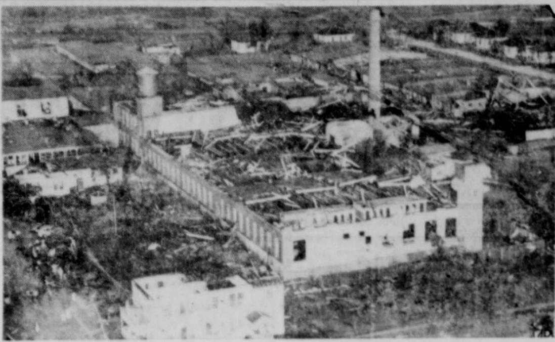
TORNADO HITS NORTH TEXAS TOWN—This air view shows the Texas Textile Mills (background) and the neighboring residential district of McKinney, Texas, which was damaged by a tornado the afternoon of May 2.
