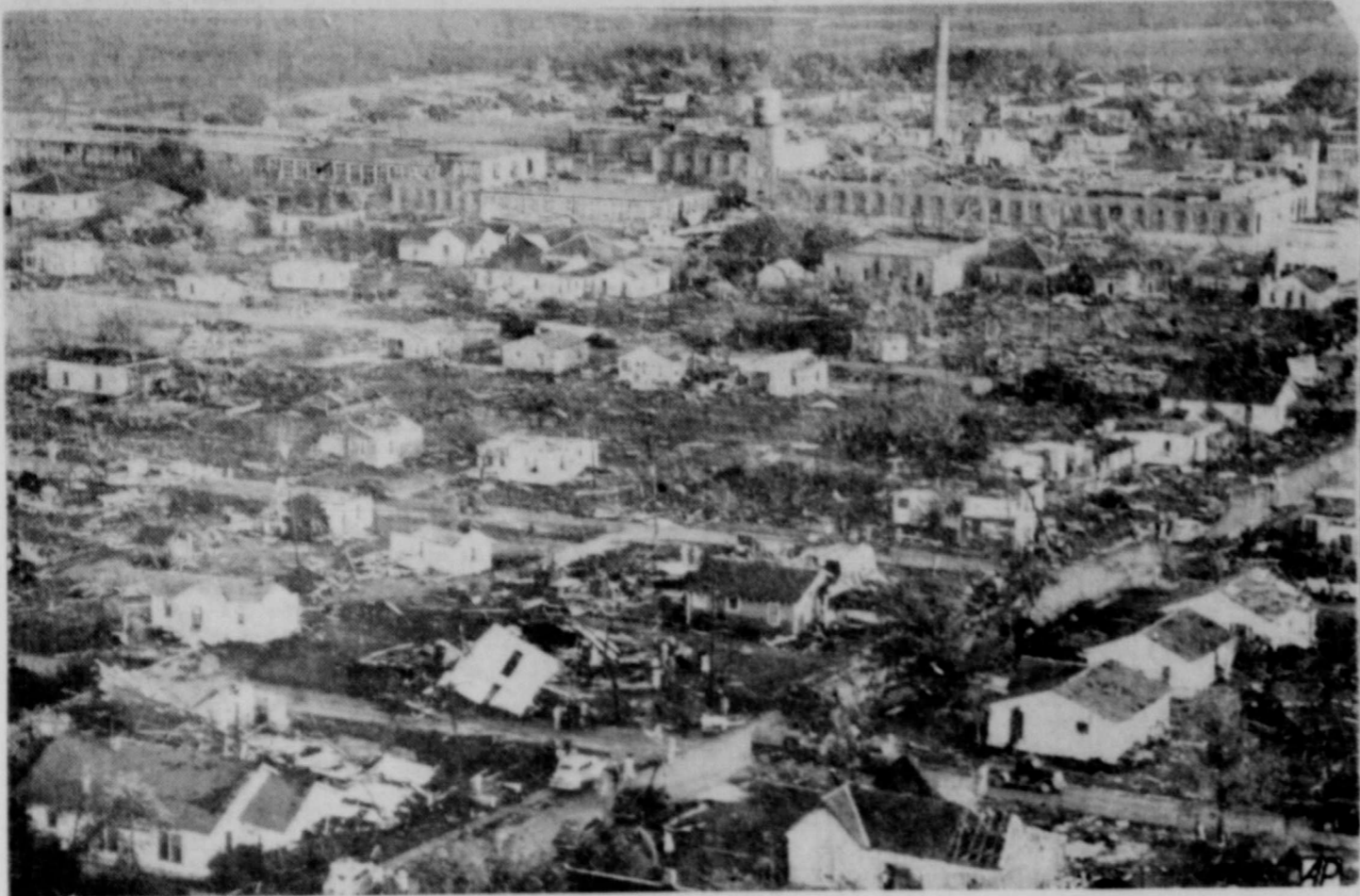
DAMAGED BY TORNADO —This air view shows the Texas Textile Mill of McKinney, Texas, which was heavily damaged by a tornado which hit the north Texas city May 2.
