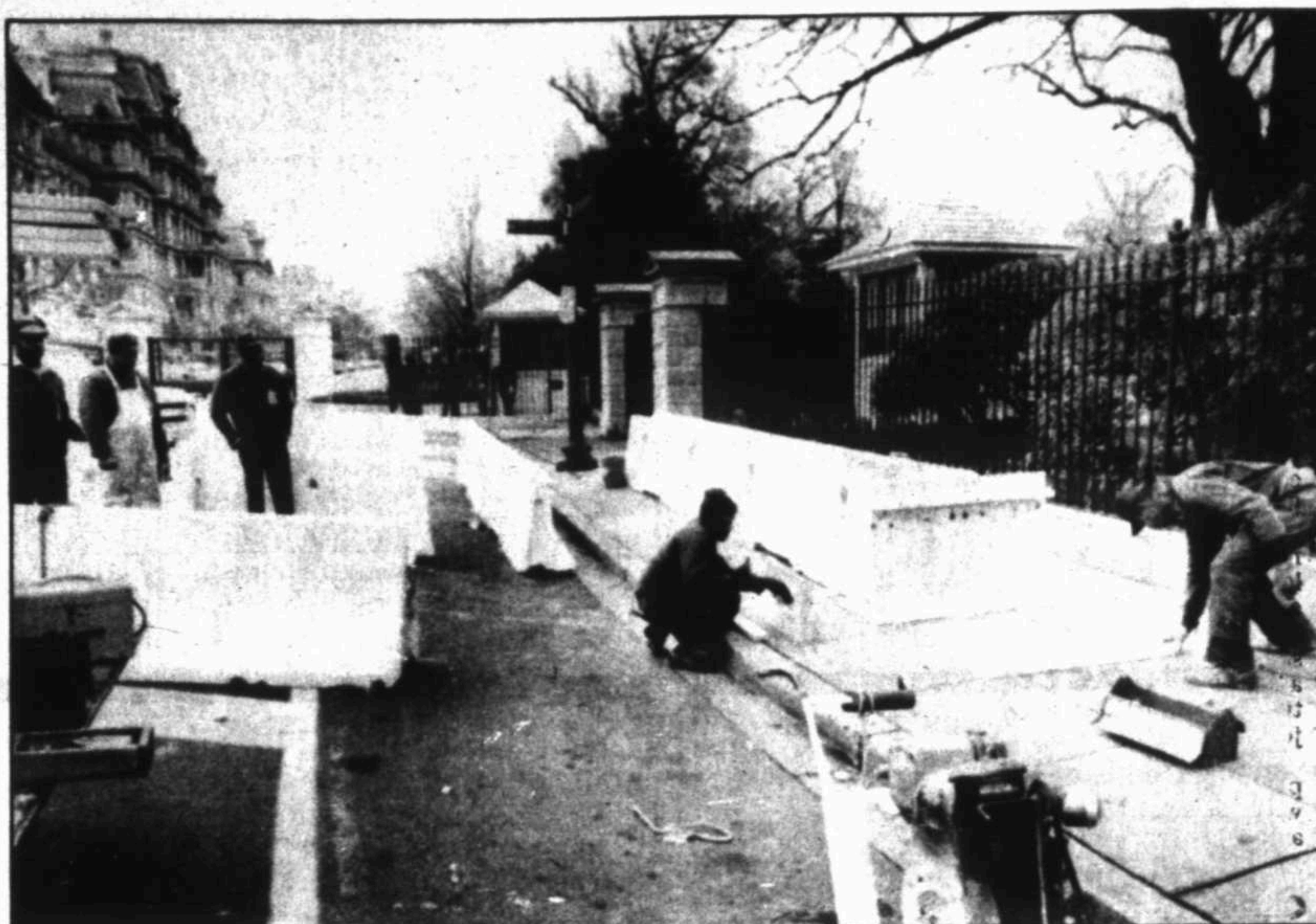
Workmen prepare 3-foot-high concrete barriers for installation at a White House gate.
