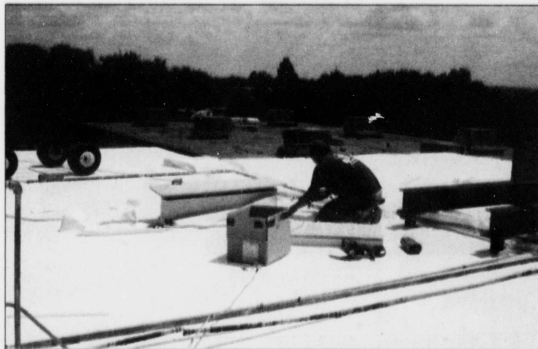
KELLEY ELEMENTARY GETS a brand new roof as Robert Sanchez secures a section of DuroLast. The single-ply membrane is rated leak-proof, wind-resistant and maintenance-free. The roofing project is part of the Qualified Schools Construction Bond grant program through federal stimulus monies. D. K. Haney Roofing, who is handling the re-roofing, will install a similar roof on the Channel 11 news building in Fort Worth following the CISD project.
