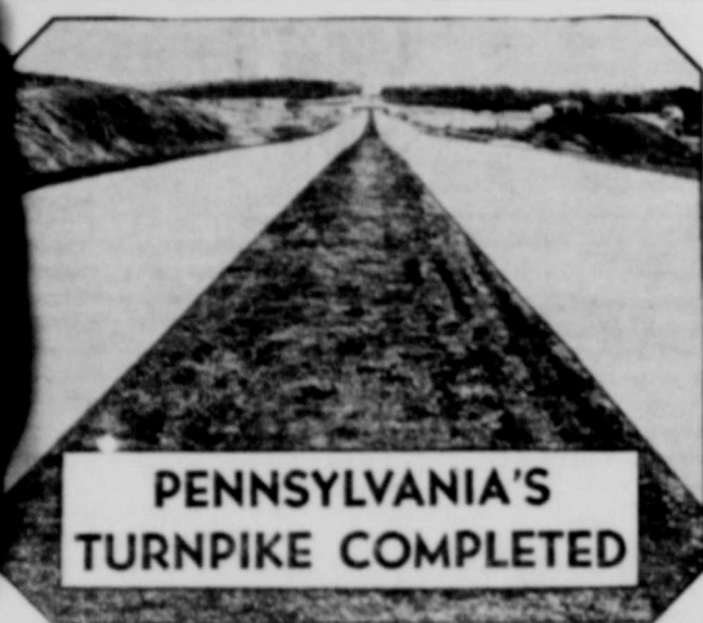
For 160 miles the Pennsylvania Turnpike stretches on like this, with few curves and no grade intersections.
