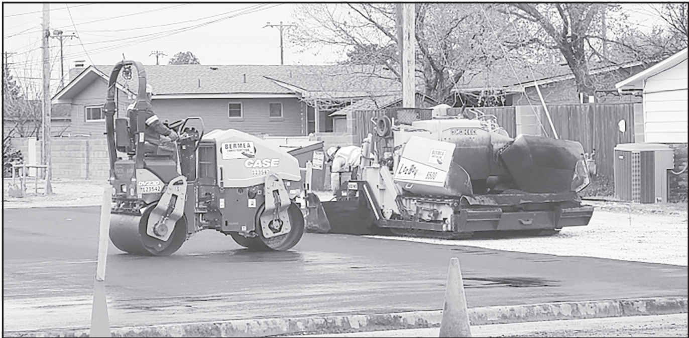
Bermea Construction paves parking lot at Bar B Studio
