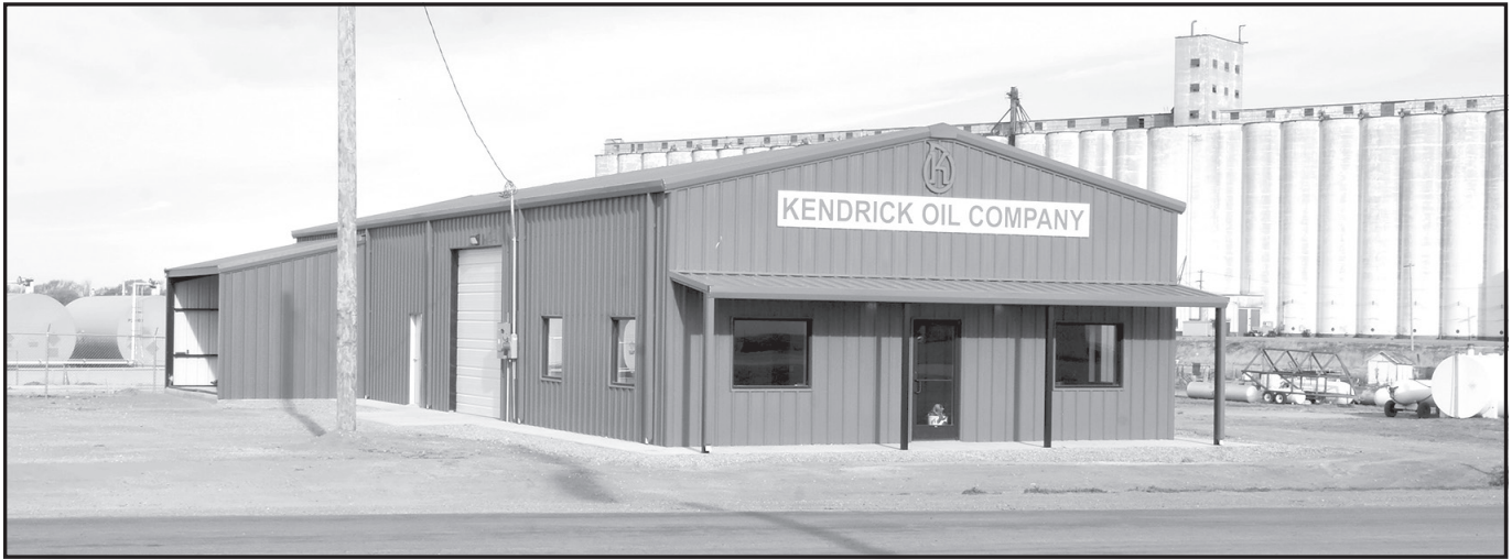
Kendrick Oil Company’s new farm store is completed
