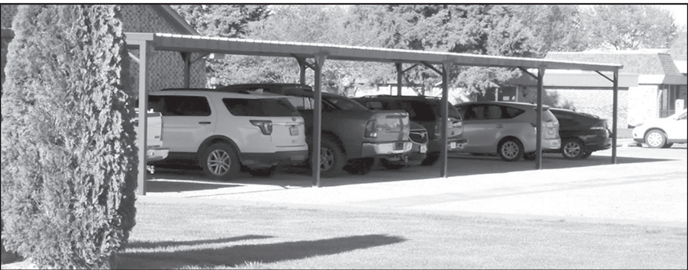
Covered carports installed on north & south side of Legacy Pointe
