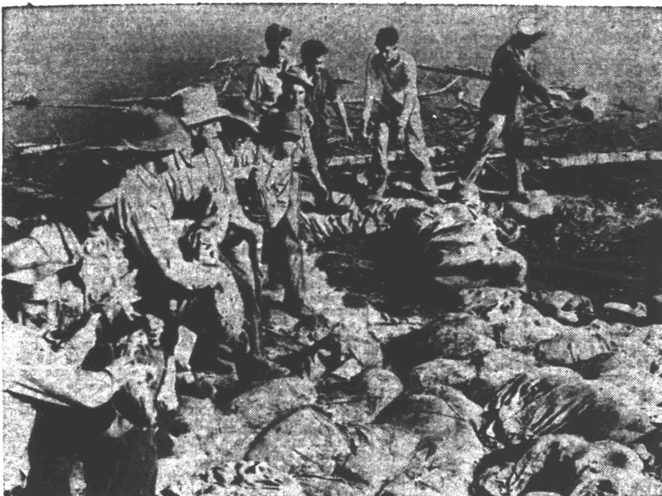
As authorities warned of a new Columbia River flood crest threatening the Portland area, workers doubled their efforts to bolster dikes. Above, flood fighters work frantically to dam rising waters with sandbags.
