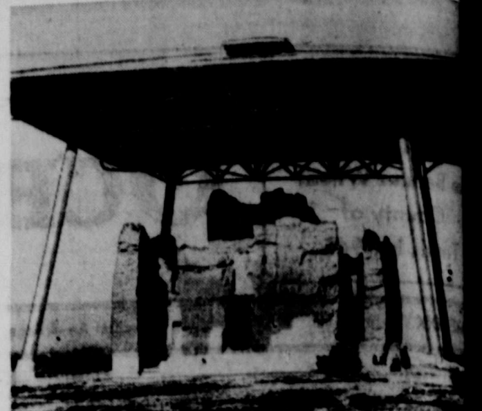
ARIZONA INDIAN RUINS —This 800-year-old ruin, Casa Grande, is one of the mysteries of the Southwest. Archaeologists have no trace of the people that built this large edifice. Today a monument, the ruins are protected by this big umbrella. The construction and wearing quality of the adobe used in this building has made Arizona residents more enthusiastic about building modern homes of this material.
