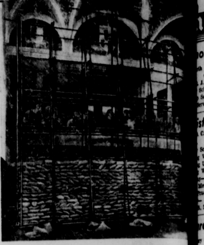
GREAT PAINTING is shown behind scaffolding when saved it in war are set up. Two nearby walls of the of Santa Maria della Grazie, site of the painting, crumbled during Allied bombing.
