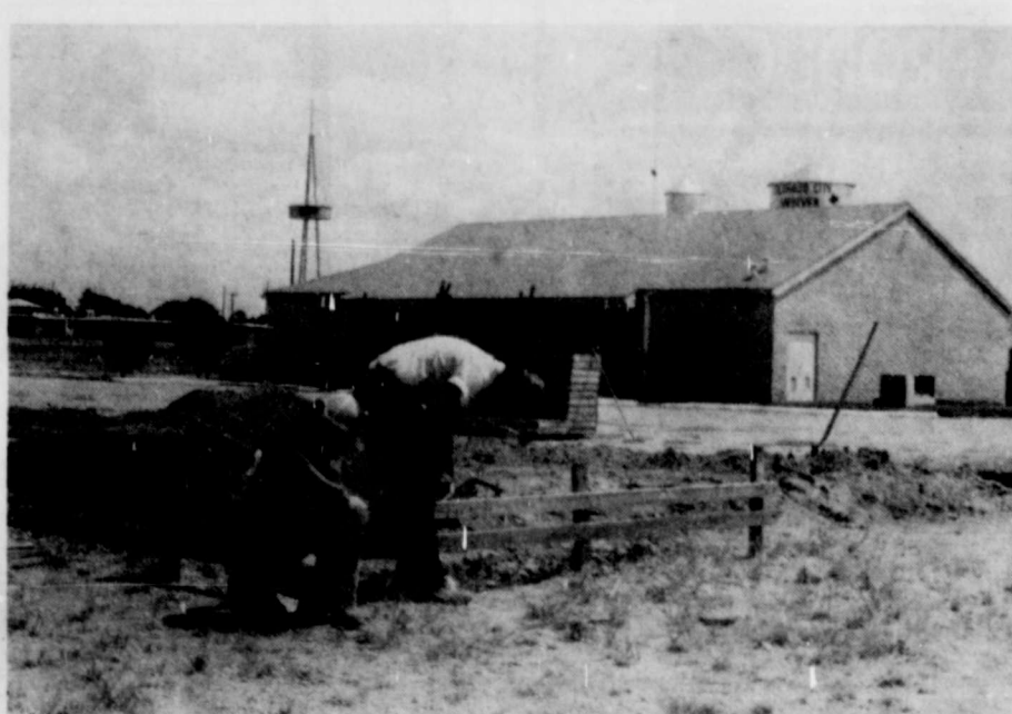
CONSTRUCTION HAS begun on a religious instruction school to be added to St. Ann's Catholic Church. According to Father John Bush, plans for the instruction school have been in the making for about two years and the school should be completed sometime next year. Cost of the building will be about $120,000 with the money coming from the parish and private donations. Religion classes from kindergarten through high school will be taught in the new building.
