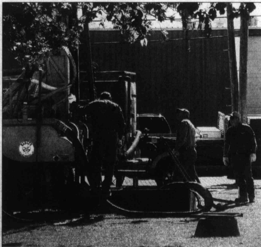
Drilling at courthouse ... A drilling rig was on courthouse grounds Monday morning, drilling a test well to gather data for a possible geothermal heating/cooling system for Lynn County Courthouse. The geothermal system is one of the planned improvements in the courthouse restoration/renovation project, to replace the old boiler system currently in use. (LCN PHOTO by Juanell Jones)
