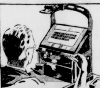
EACH "HEAT" OF ALLOY IRON AND STEEL MADE IN THE FORD ROUGE FOUNDRY IS ANALYZED BEFORE IT IS POURED BY TAKING PHOTOGRAPHS OF THE SPECTRAL "RAINBOWS" FORMED BY ITS ELEMENTS
