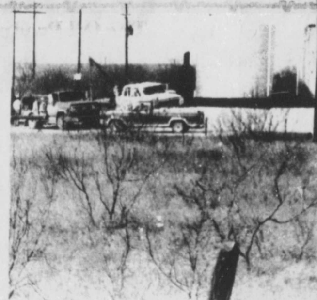
Wells Must Be Serviced
