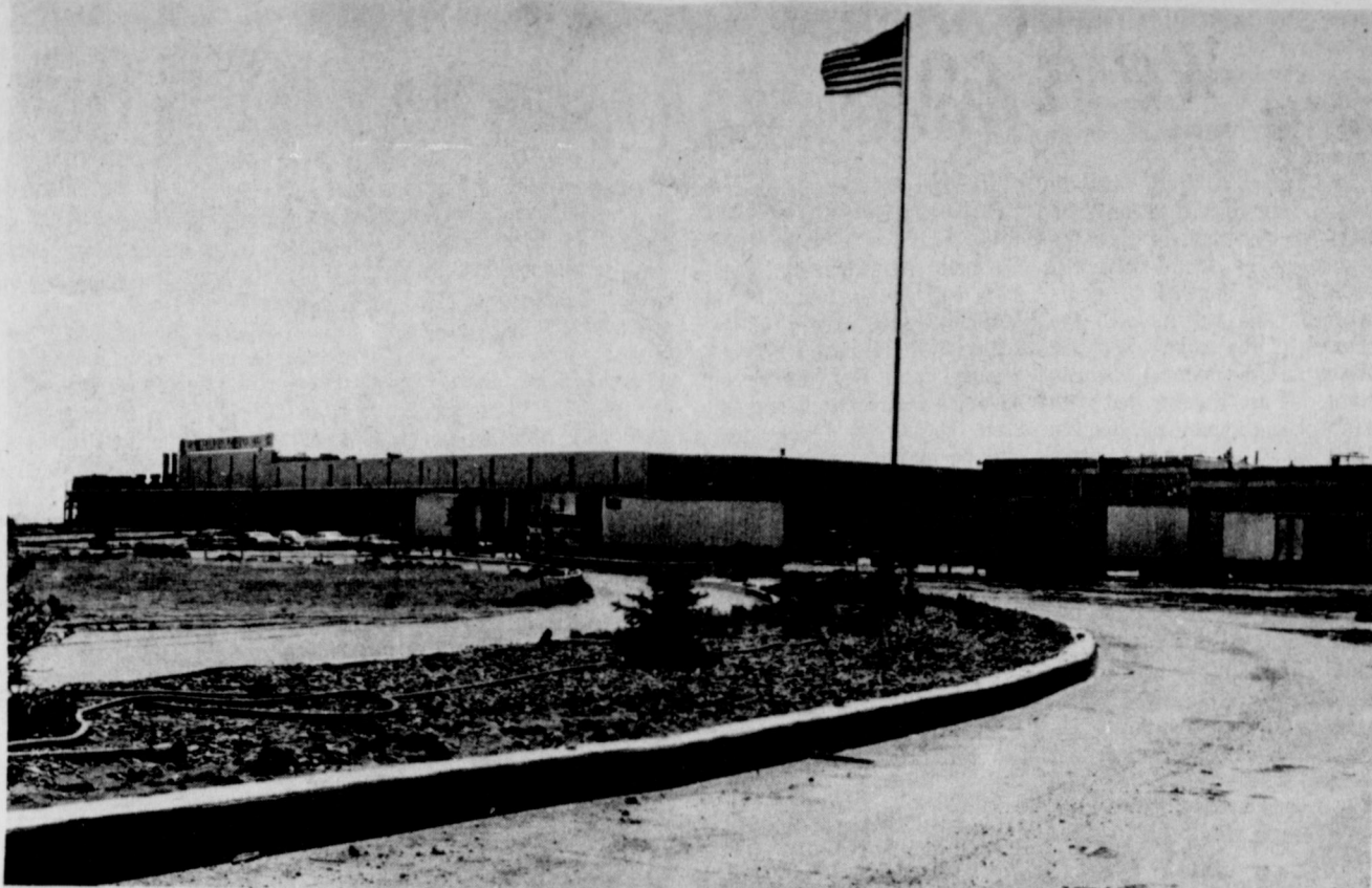
HEAVY DAMAGE TO MISSOURI BEEF -- Around $50,000 damage was reported by Missouri Beef Packers at Friona following a tornadic windstorm which hit the plant late Friday afternoon. Although members of the press were not allowed to go past the guardhouse at the gate of the huge plant, workmen were noted
