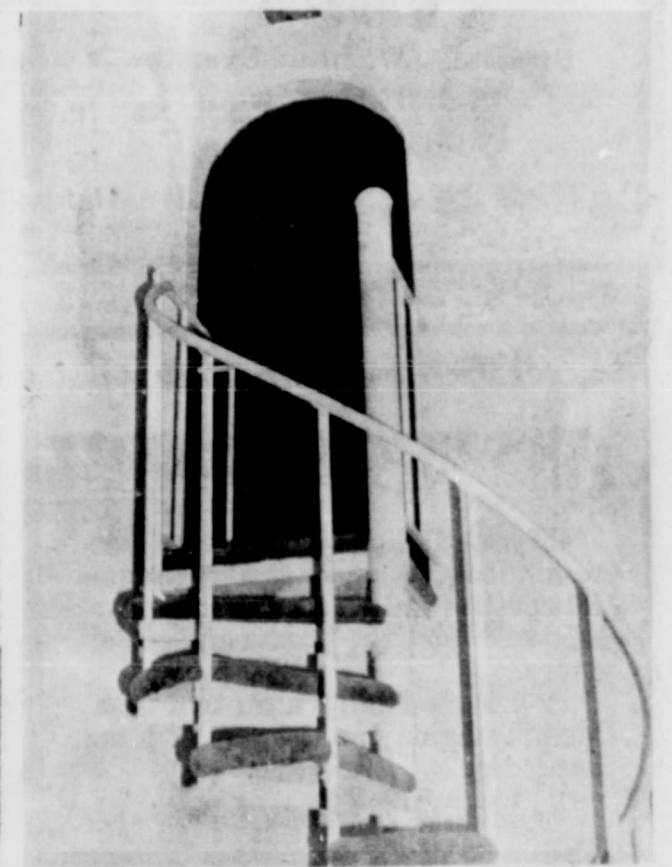
Staircase To Loft
