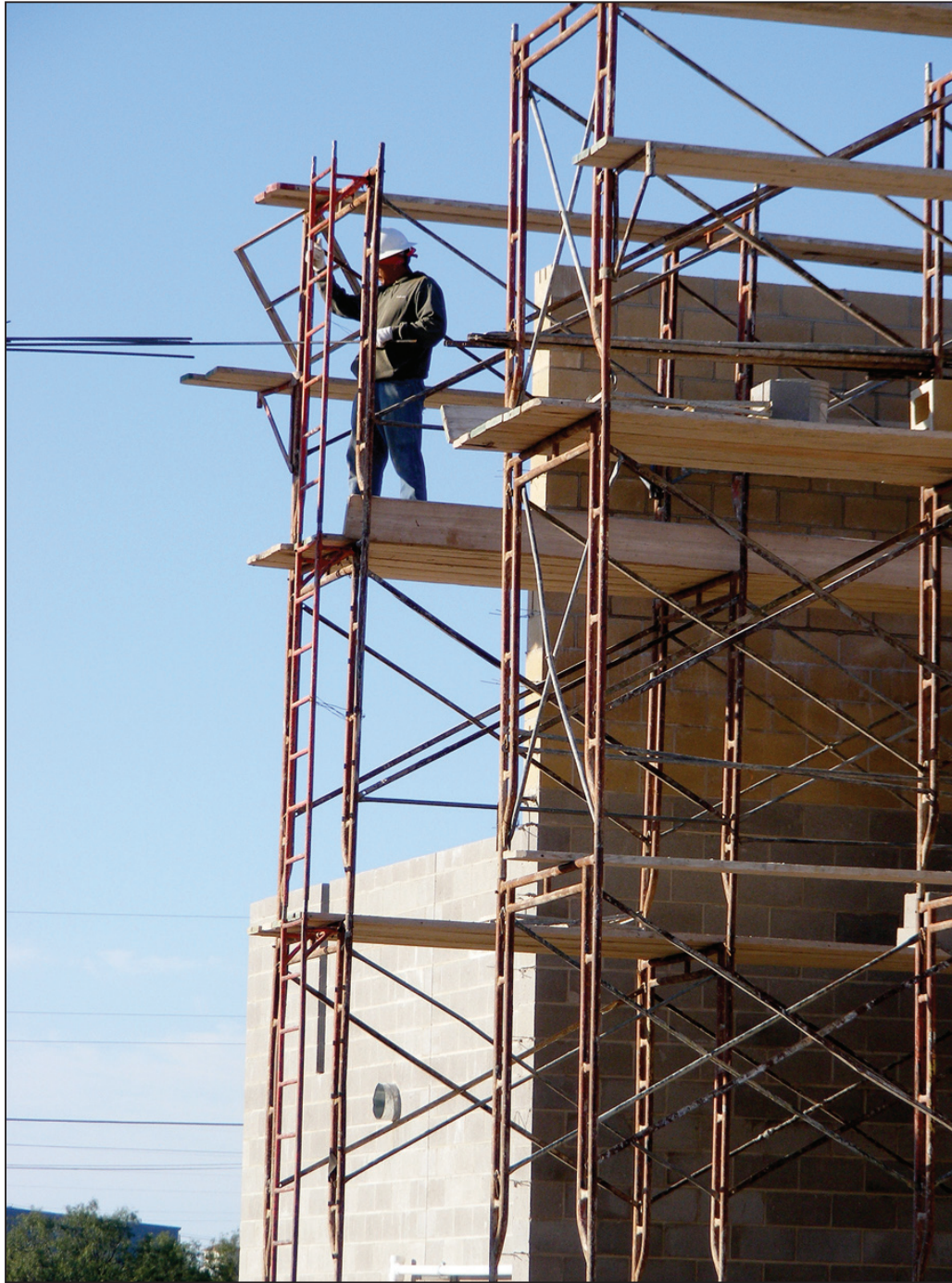
HERALD photo/Steve Reagan A worker unloads reinforcement bars off a pallet at the site of the future Howard County Jail on West. Highway 80. Construction on the jail, which began in earnest this summer, should be completed by mid-2009.
