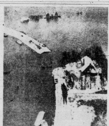
BREAK IN DUTCH DIKE —Water pours through a break in the North Sea Canal dike at Oost-Zaai, Holland, forcing some 10,000 people from their homes in the Westerdijk suburb. Damage was estimated at about $1,300,000 (AP Wirephoto).
