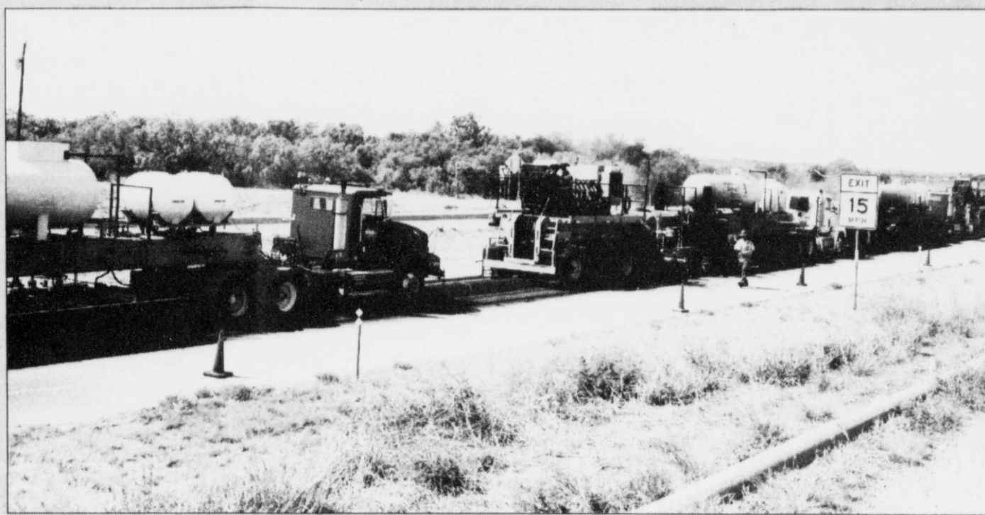
MOVING RIGHT ALONG a construction train heats, chews up and flattens existing pavement into a smooth driving surface along Interstate 20 in Mitchell County. The innovative technique by Dustrol Inc., is a 100% recycling process, the first of its kind in Texas.
