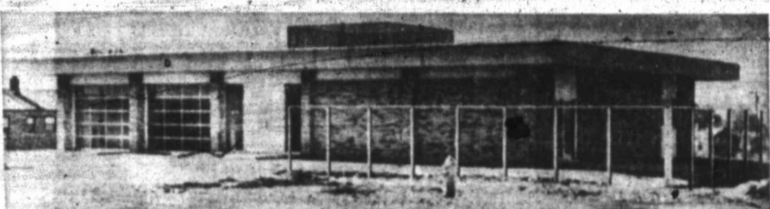
AIRPORT ADDITION STATION Located at 2906 W. 13th
