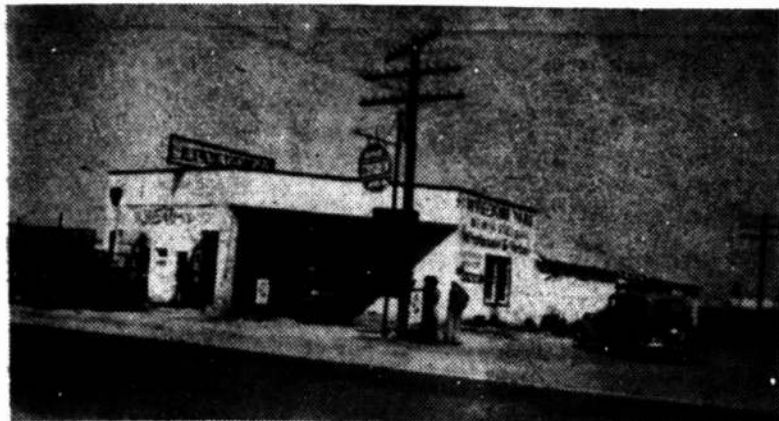
Out-door view of Lamesa Salvage Shop, owned and operated by Elmo Smith, enterprising business man of Lamesa.
