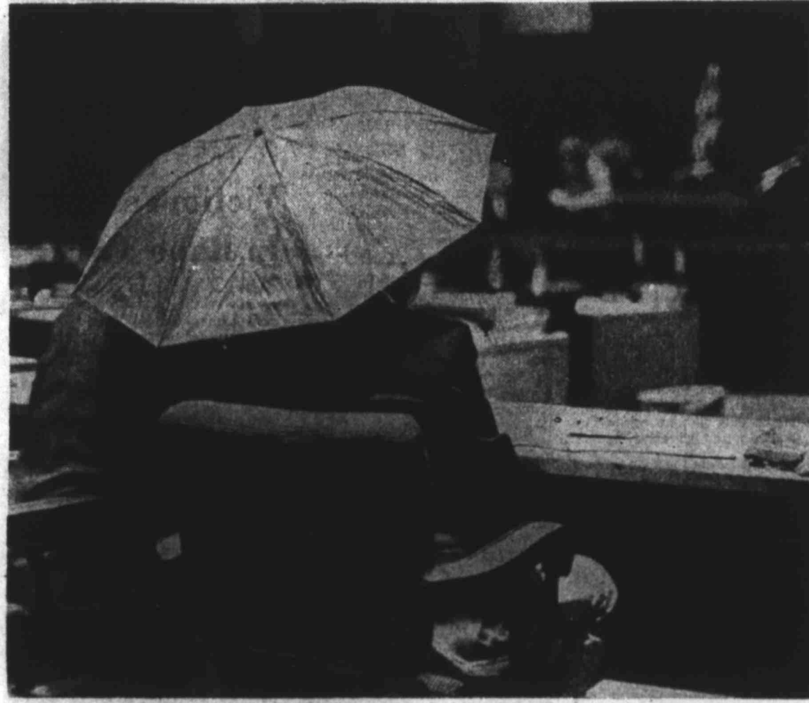
RAINDRIPS KEEP FALLING — Legislators Larry Bahill, D-Tucson, and Larry Hawkes, R-Tucson, use an umbrella for protection after the roof of the Arizona House of Representatives started leaking Wednesday. The leak did not interrupt business, although it did cause some solons to evacuate their damp seats and move to dry locations. (AP Laserphoto)
