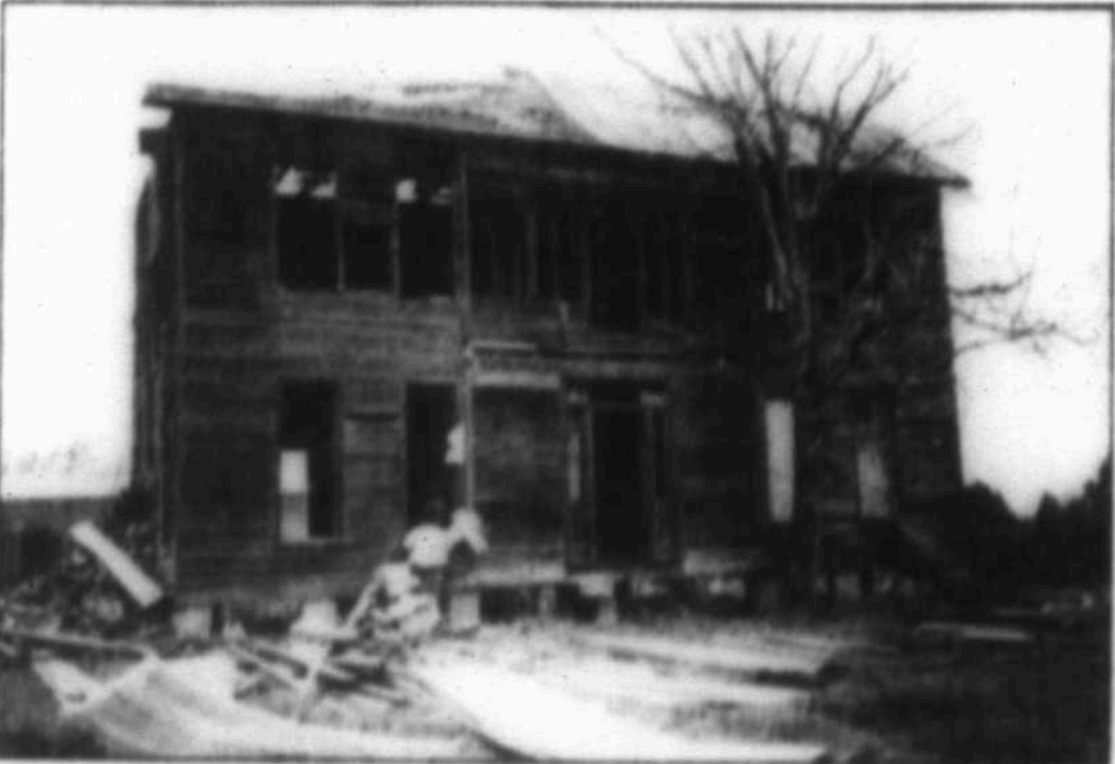
Workers dismantle an old house in Milano and will use the aged cedar boards to build a United Pentecostal Church that now conducts worship services in the back of a Rockdale store.
