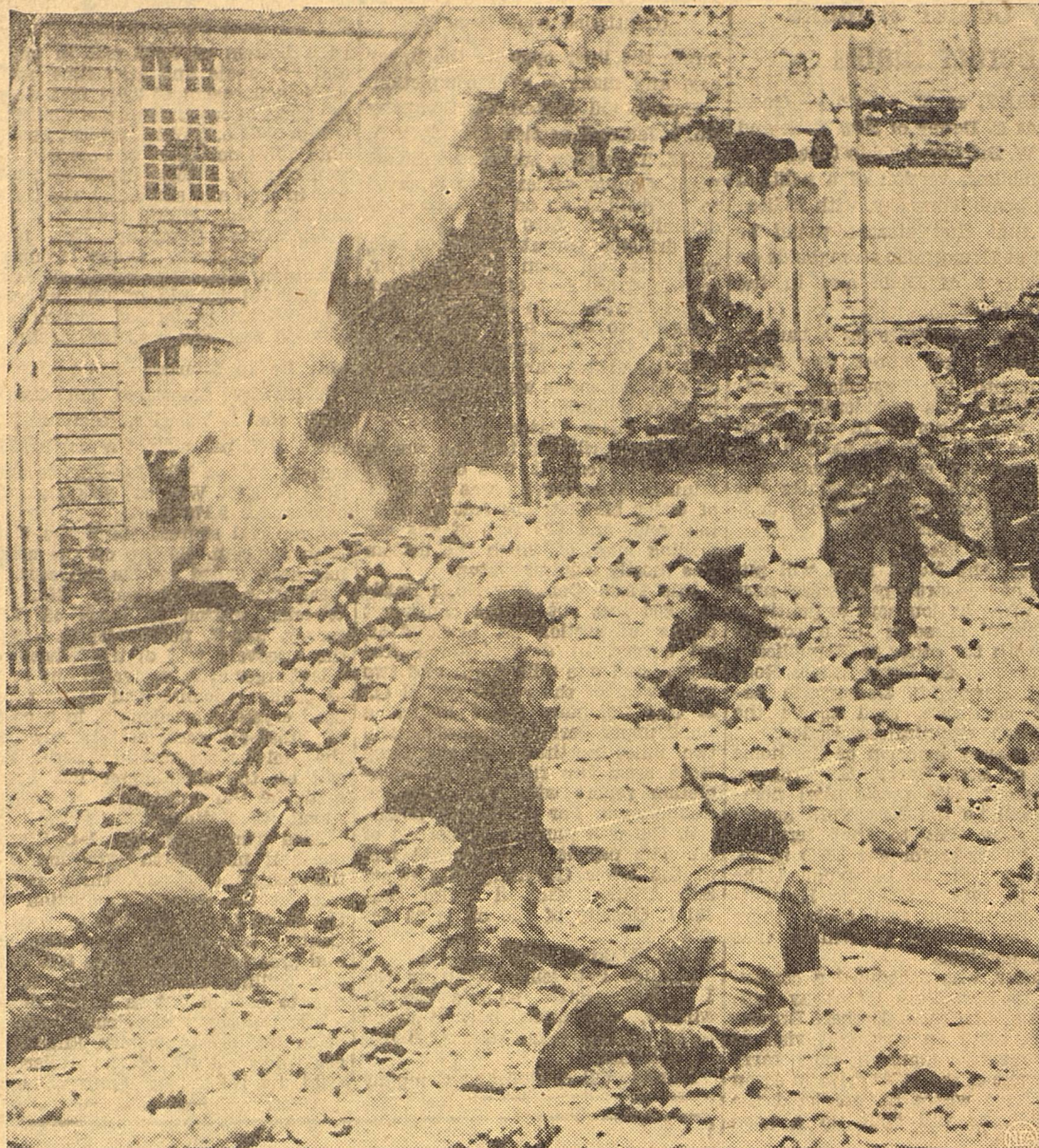
The remarkable action photo above shows what Yanks were up against in capturing La Haye du Puits, on Cherbourg peninsula, where Nazis were well entrenched. Germans holed up in a chateau are being blasted out. Note front wall crumbling from grenade or shell explosion. Yanks in photo prepare to rush the position, two of them dashing forward under covering fire from their comrades on the ground.
