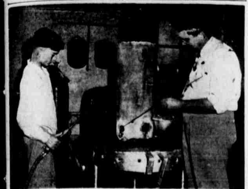
FFA SHOP PROJECT —Shown above is the welding section of the workshop of Post high school's chapter of Future Farmers of America. Donald Mason, left, is receiving instructions from E. F. Schmiedt, vocational agriculture teacher, on correct method of finishing the welding job on his automatic water trough for his swine project. This water trough is one of the many shop projects completed by the FFA members during the first three months of the 1952-53 school term.—Dispatch Photo
