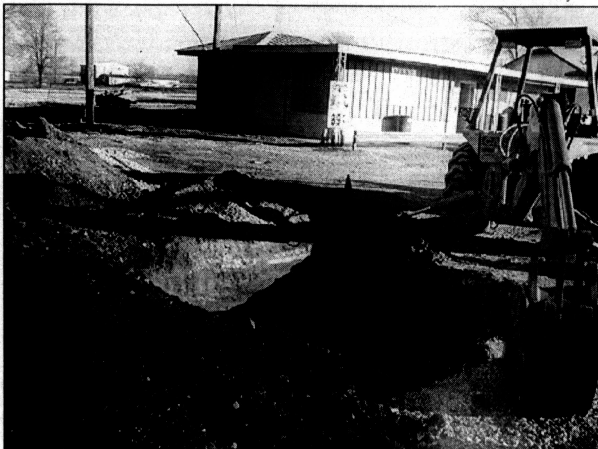
THE CITY OF LORAIN WATER DEPARTMENT installed 11 new water main valves last Friday, causing the town to be without water for more than 12 hours. The one pictured is in front of Maz's Place. Ricky Bailey, Water Superintendent, thanks all the citizens for their patience during the water outage.
