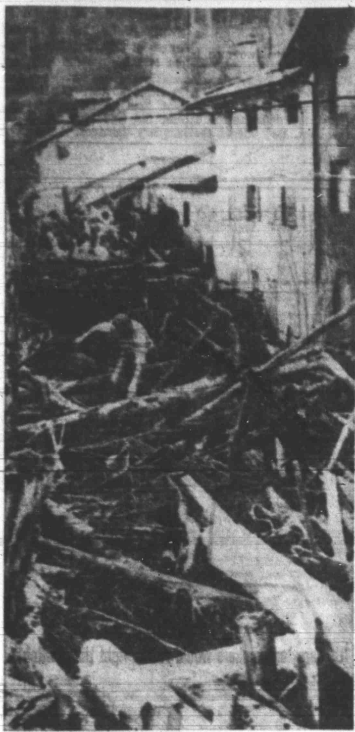
Clogged Italian Street
