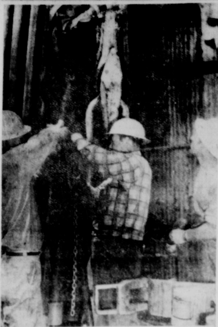
INSERT SAFETY PLUG —Members of the McGarrugh No. 1-B crew are shown placing a safety plug in the drill stem in preparation for Tuesday's drillstem test. Shown from left to right are J. D. Conners, driller; A. M. Herring, motorman; D. Moss, floor man; and C. M. Rozell, (above) floor man.
