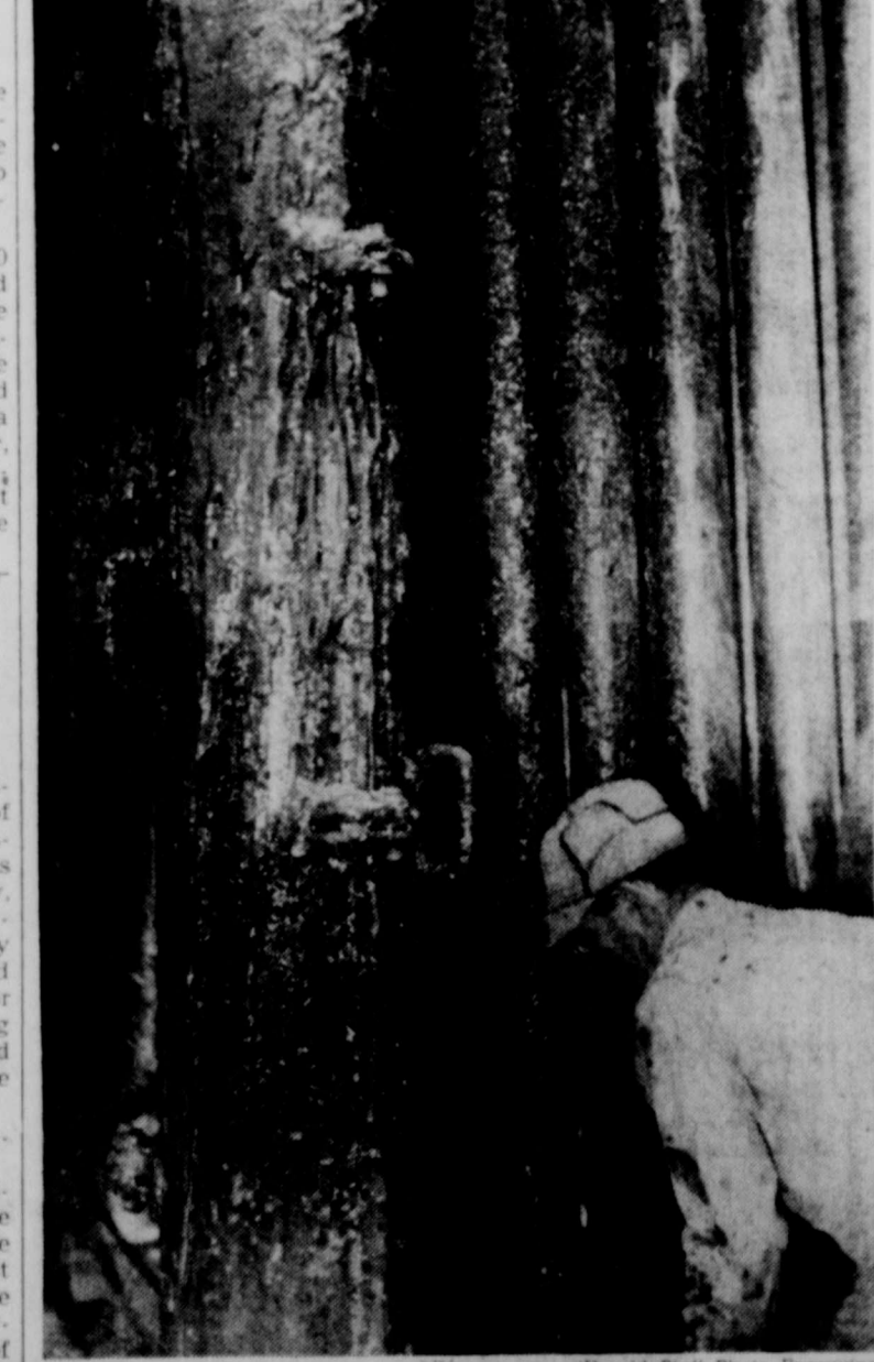
IT'S OIL AT MCGARRAUGH 1-B—Oil and gas cut mud flows from the top of the drill stem in Tuesday's test at McGarraugh No. 1-B where 38.7 oil was recovered in the county's petroleum show. Joe Foster, Halliburton formation tester from Perryton, is shown securing a sample.
