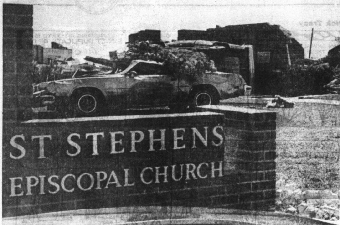
St. Stephens Episcopal Church on Cypress was demolished
