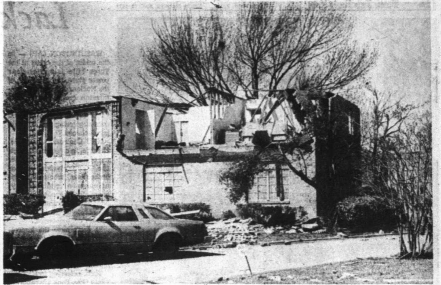
Southmoor Manor apartments damaged
