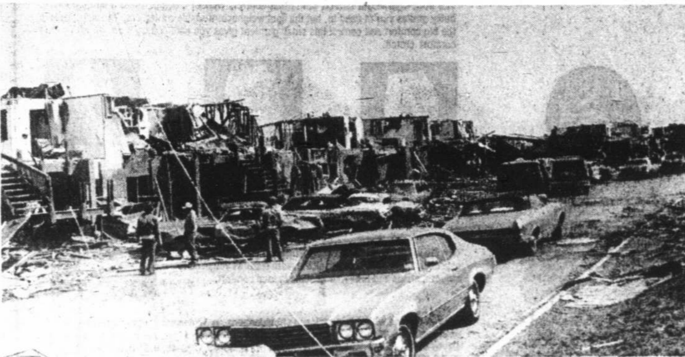
Damage was heavy at apartments
