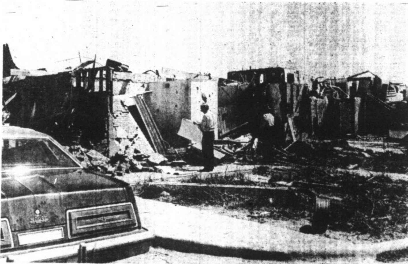
Insurance adjusters inspect damage
