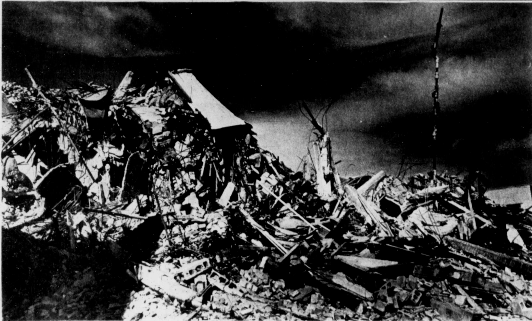
SOME MIDLANDERS consider the ongoing demolition of the old Llano Hotel building at the corner of Wall Avenue and Main Street to be the best show in town right now. The con-
