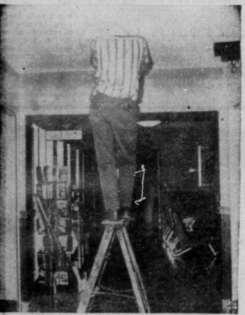
OUT OF SIGHT — This workman went through the ceiling when told to fix a light fixture. Scene took place in the lobby of Memorial Hospital in Albany, N. Y.
