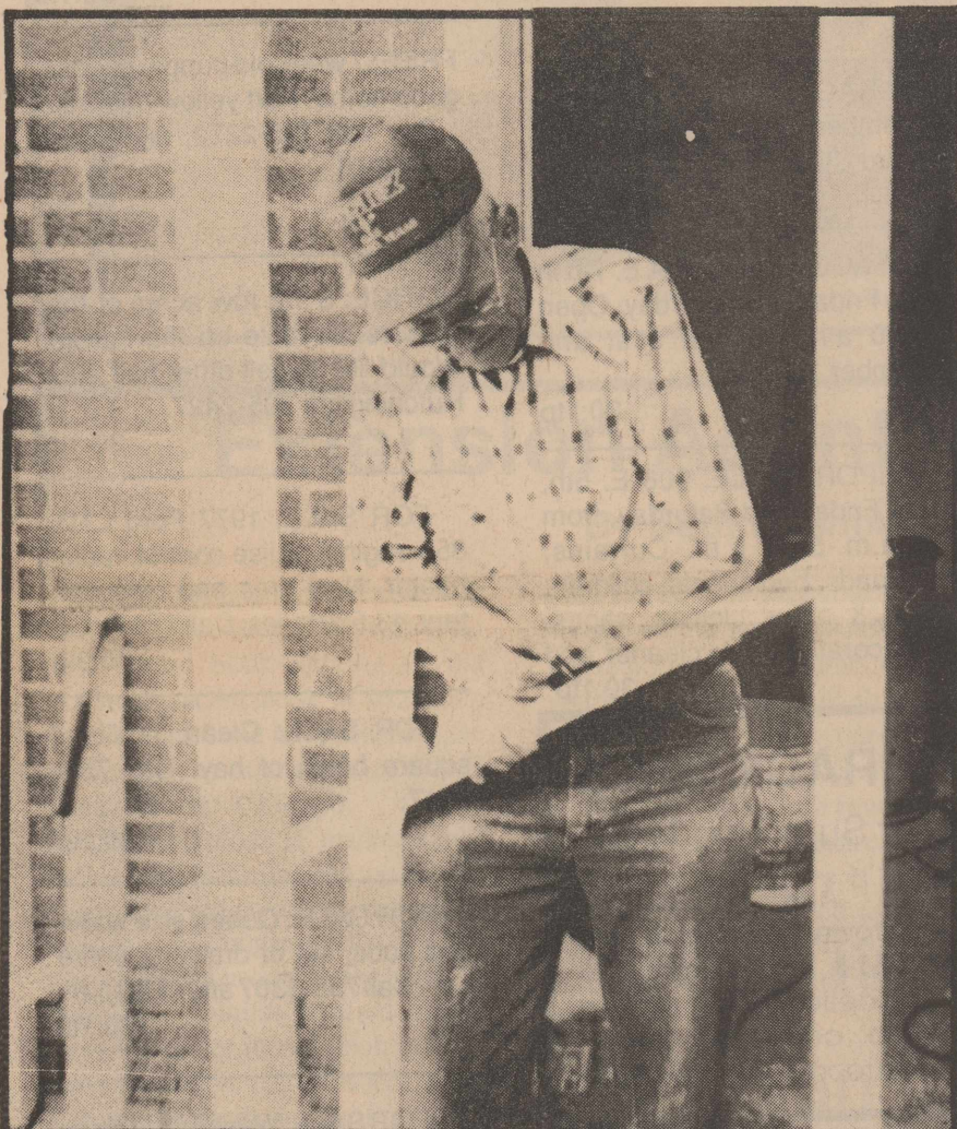
BUSY AT WORK: Alvin Seaton, Roby School Maintenance Department, was busy at work finishing a new addition on the Roby Elementary School building, last week. Seaton was constructing restroom facilities for teachers.
