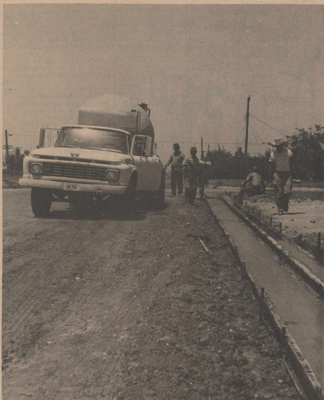
PAVING UNDERWAY--Workmen from High Plains Pavers from Plainview are shown as work got underway this week on a city paving project that will take in approximately 18 blocks. The construction will take approximately six weeks if weather stays fair.
