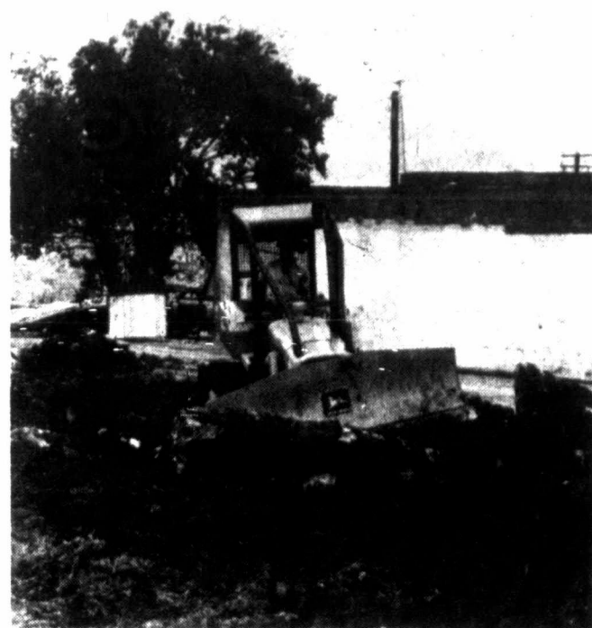
GROUNDS FOR a gazebo and city park are being prepared as rocks and earth are moved by Ben Sparks Construction crews. Sparks donated labor and equipment to expedite construction of the gazebo and park area. Wallace Center originally began the gazebo project plan with a Levi Strauss Co. grant. A lot, located at the corner of Chestnut and Second Streets, was donated by Dell Barber to the Kiwanis Club. They, in turn, donated the property to the City for the park site, which will include the gazebo and a lighted water fountain. Completion of the project is anticipated prior to the Centennial Week Celebrations in July.
