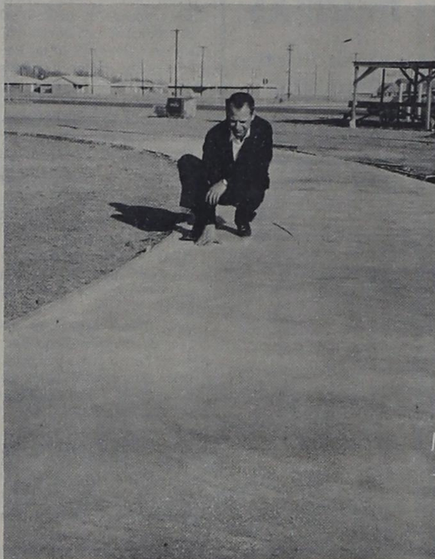
NEW RUNWAY -- Edward Isaac, a member of Bovina Modelers, is shown inspecting new concrete poured last week for a runway for Bovina's model airplane port. The new facility will be initiated during Sunday afternoon's 100-mile rat race in which some 20 contestants are expected to enter. The circular runway was constructed with members of the organization doing the labor.
