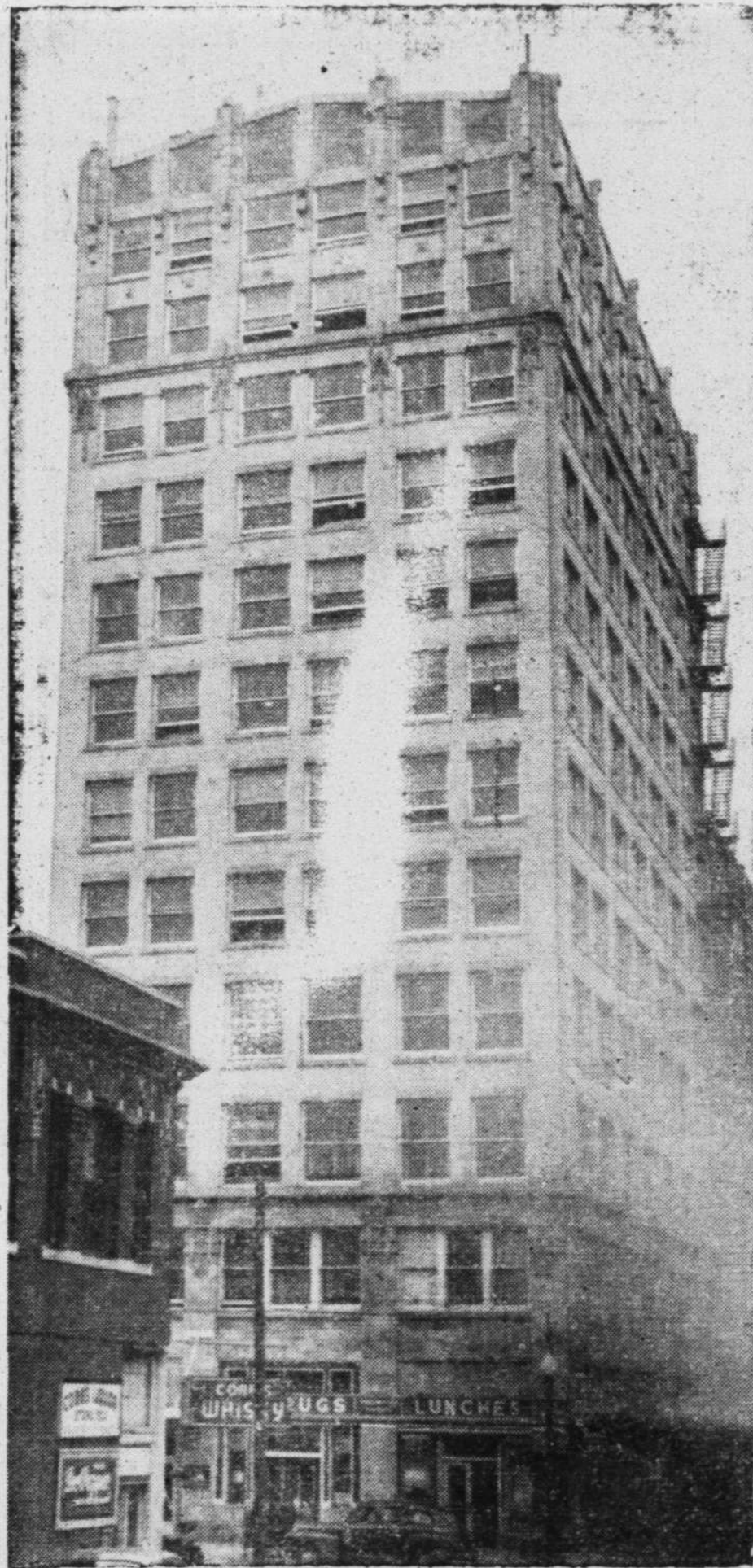
This entire 12-story office building in Dallas has been requisitioned by the Federal government to house agencies designed to speed the war effort. Tenants of the building, known as the Fidelity Building, were asked to vacate as quickly as possible.
