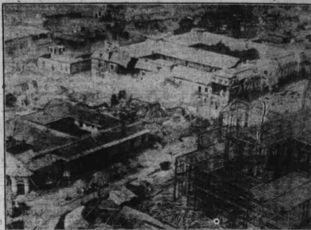
The smoking ruins of Managua, Nicaragua, are shown in this air view of the city taken while flames consumed wreckage left by terrific earthquake shocks. How buildings were leveled by the quake and walls shattered is shown by the photo. The death toll is expected to reach 2,000 while property damage was so heavy it is doubted if the city will be rebuilt.
