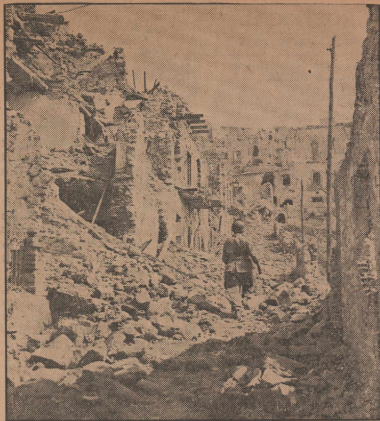
NO WONDER THE GERMANS LEFT! The pounding taken by Castleforte, Italy, in the new Allied offensive is grimly evident here as an American soldier picks his way along a rubble-strewn street. Not a building looks salvagable.
