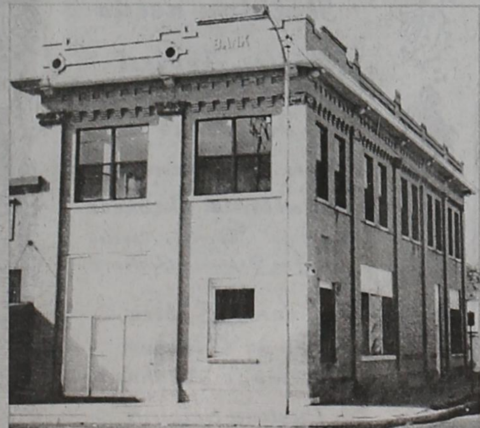
Historic building being restored
