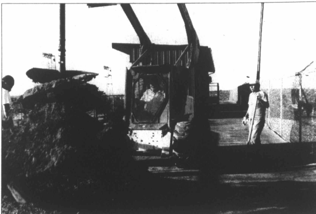
LIGHT IT UP! Longhorn Electrical employees (l-r) Jason Davis, Johnny Bankston and Ernesto Ramirez dug the holes for the new light poles at Wolf Stadium. The six old lighting poles on the home side are being replaced with four new 70' poles.
