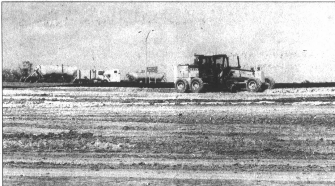
HITTING THE GROUND RUNNING — Dirt work has begun in earnest on the future site of the Lone Wolf Creek RV Village, east of town along I-20. Plans for the property include RV spaces with a lodge-type atmosphere.
