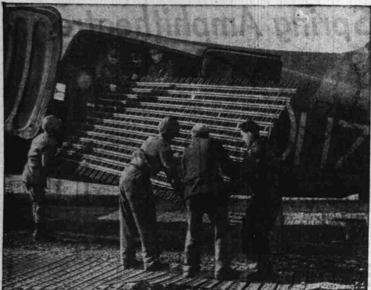
RAF CARRIES OWN RUNWAY —Ground crewmen unload a 6 by 12 foot strip of metal runway from a Dakota plane of the transport command as RAF takes over a Belgian base.
