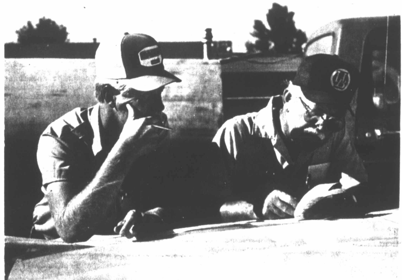
TAKING INVENTORY — Mark Patterson and George Lee inventory the supplies needed for waterline construction along 37th St., a project that began earlier this week. (Howard Bigham Photo)
