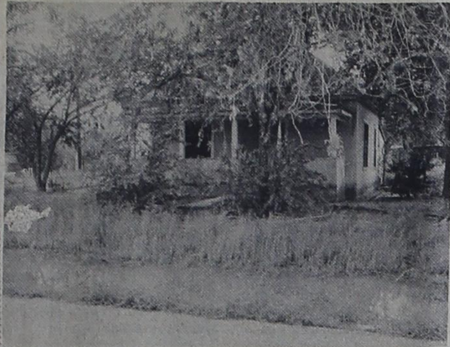
The battle by city fathers to rid the town of mosquitoes is a losing one until owners of vacant lots and houses such as these clear away the unsightly weeds which have grown rampant making ideal breeding places for the mosquito population. Pictures one, two, and three show houses which could be made into nice dwellings, if the weeds were cleared away; while picture
