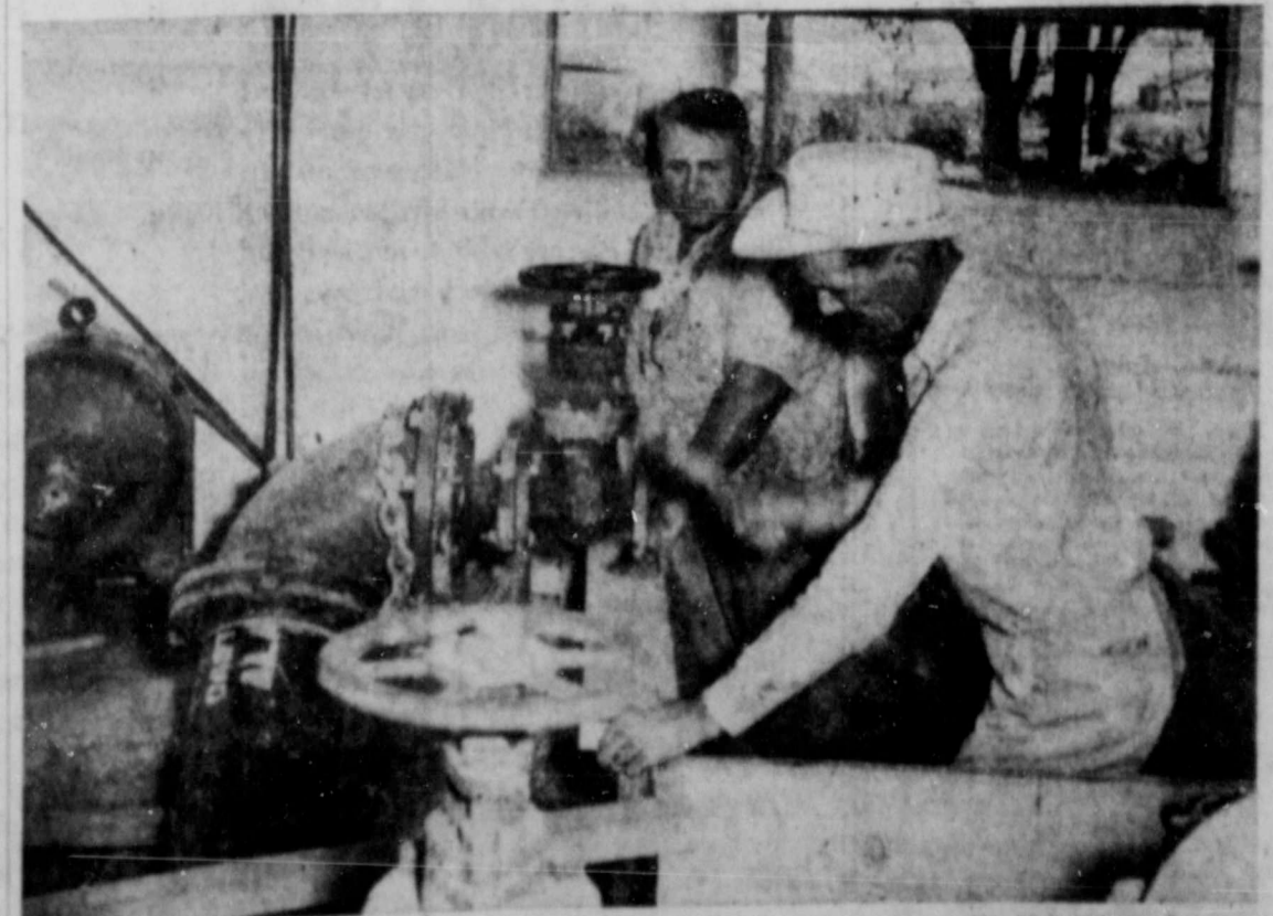
BOOSTER PUMP—Harold Bryan and Elza Kutch, city employees, are shown preparing to install the booster pump for the new city water well. This pump, installed at the city park well house, will pull water from the well into the city tower, boosting city water production for the hot days that lie ahead. See No. 4, Page 6
