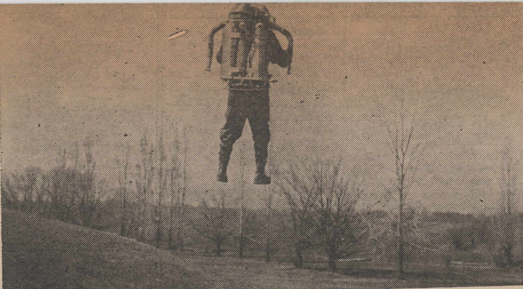
NO VISIBLE MEANS OF SUPPORT — Bell Laboratories engineer Harold Graham becomes the first man to fly a back-pack rocket. He rose 30 feet into the air in Buffalo, N.Y., and wooshed over the ground for about the distance of a football field.
