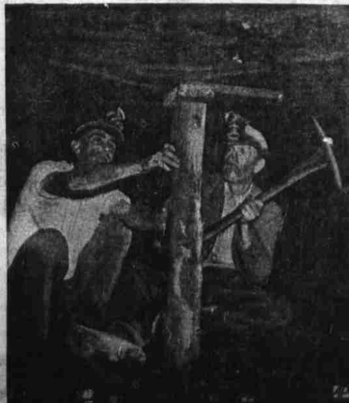
TRIAL OR NO TRIAL , Harlan miners keep on working while workers' testimony of alleged intimidations go into the court record at London, Ky., trial. Down in the mine, Jay Depew (left) and "Uncle Ben" Spurrlock brace up ground.
