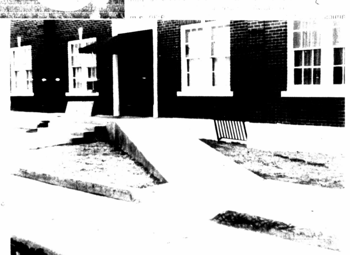
HANDICAP ACCESS —A ramp incline, providing easier access to the City Hall by handicapped and elderly persons was constructed the past week. Numerous modifications are also being made inside the City Hall to meet handicap access regulations.
