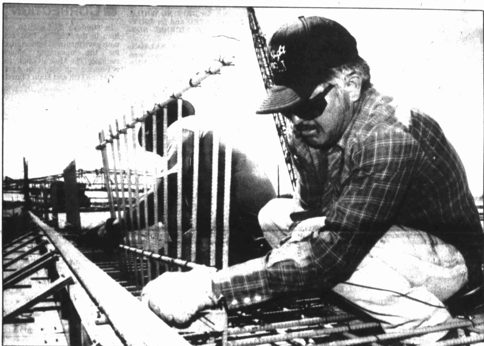
Construction workers tie a steel frame into place where a concrete guardrail will be erected as work continues on the westbound Interstate 20 bridge near FM 700 Wednesday. The bridge is nearing completion, with the eastbound bridge scheduled to be demolished and rebuilt.
