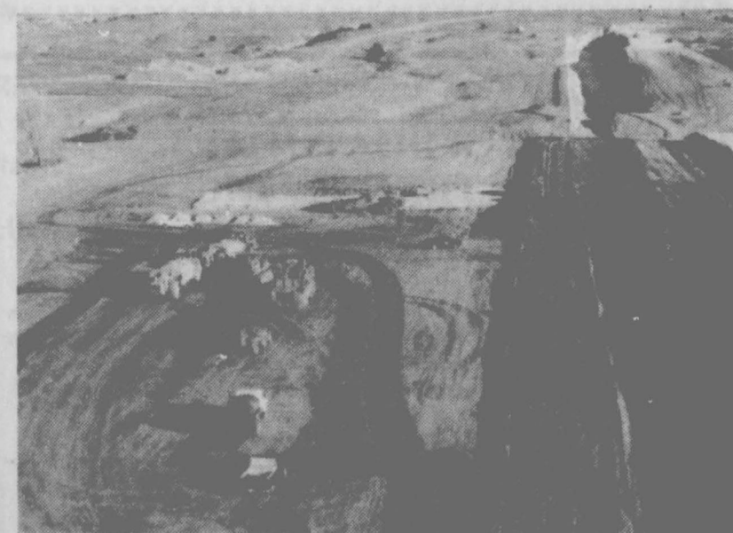
Construction workers at the Palo Duro Dam site have accomplished a lot lately. The weather has been cooperating so far. Visitors are encouraged to come to the overlook and see how much has been done.
