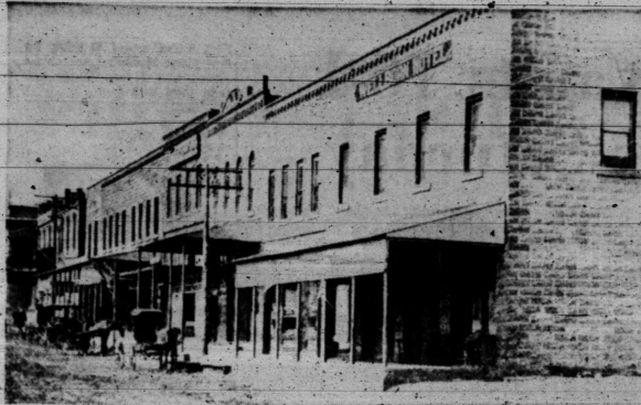
BUILT SEVERAL YEARS BEFORE the present courthouse, this building at Twenty-fourth Street and Avenue S was used as a hotel up until recent years. It is pictured about 1908 when for a brief time it was the Wellborn Hotel after the original Wellborn burned. It soon became the Woodrow Hotel under which name it operated for many years. The building was built in anticipation of the boom which followed the railroad's arrival in 1908.
