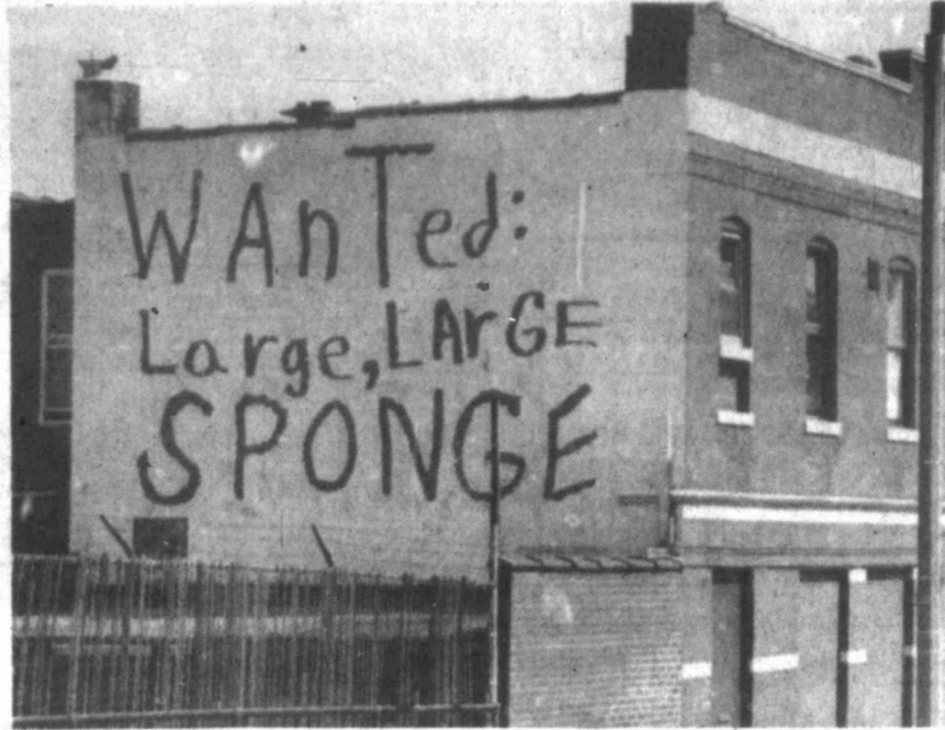
At left, a homemade message on the back of a St. Louis building shows some humor among the sometimes sudden sentiments created by the Midwest flood. At right, the fingers of Mark Roth are bandaged, covering up blisters earned from days of filling and tying sandbags in St. Genevieve, Mo. The rising waters of the Mississippi River are forcing residents of this historical town to work around the clock in an attempt to save their property.
