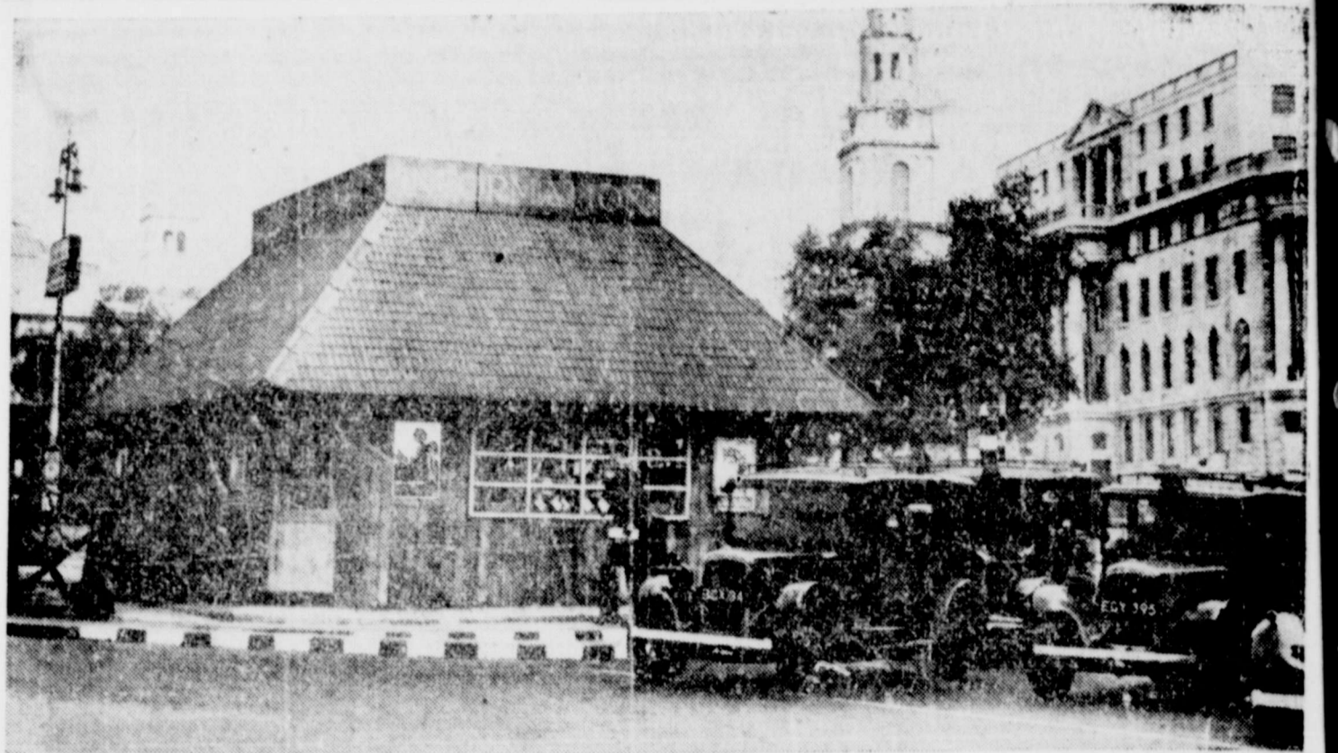
LONDON DISMANTLES —With fear of Nazi invasion lifted, London dismantles pillboxes and strongpoints built in 1940 throughout city. Above information booth which appeared overnight in Trafalgar Square on site of King Charles statue is really concrete reinforced strongpoint protecting approaches to Whitehall, Buckingham Palace, and the Strand. In background are St. Martin-in-the-Fields Church and South Africa House.
